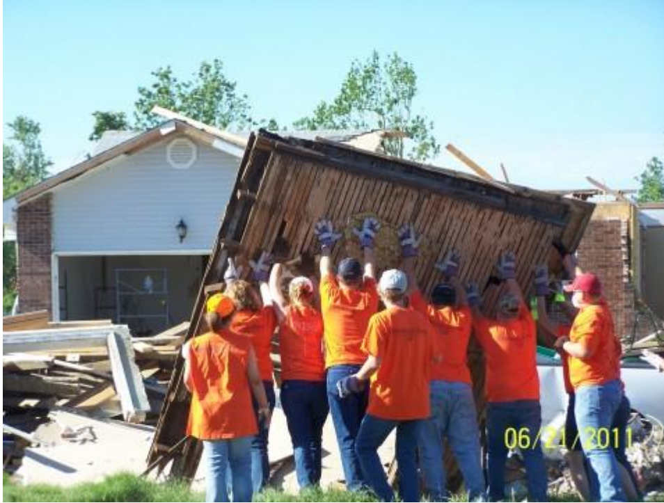
Disposing of a wall.
